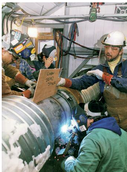
大口径双相不锈钢跨境管道的机械化焊接 © Arco Exploration and Production Technology
